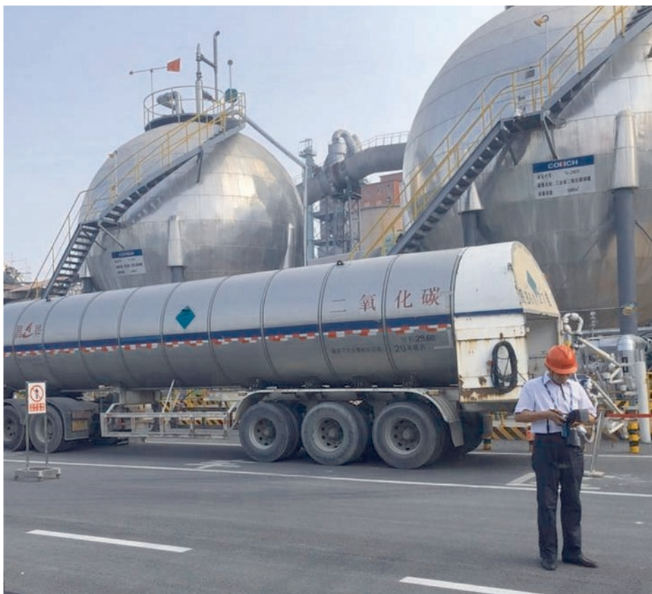
CO 2 storage vessels, and a lorry being loaded with liquid CO 2 for transport to the usage endpoint at the Conch Wuhu CCUS facility in China. The Baimashan Cement Factory in Wuhu uses amine technology to capture CO 2 from its cement kiln
