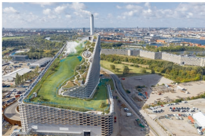
ARC is investigating the possibility of capturing CO 2 from the Amager Bakke waste-to-energy plant in the city of Copenhagen (Photo: Amager Resource Center/Ehrhorn/Hummerston)
